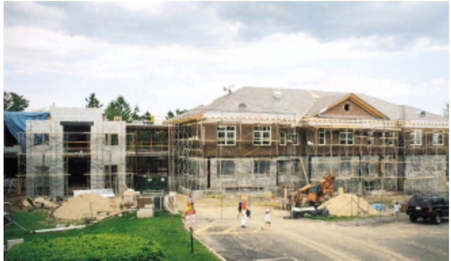
The Eileen Dealy Gillespie '49 Science Center under construction in 1998.
